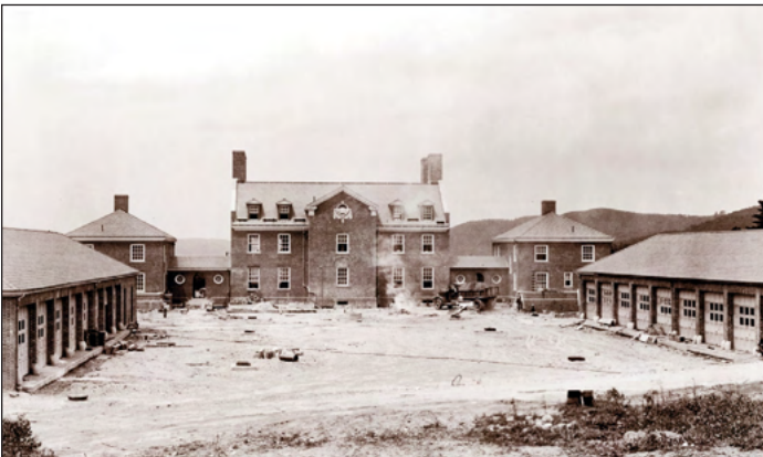
View of administration building, annexes and garages from the rear - July 1938
