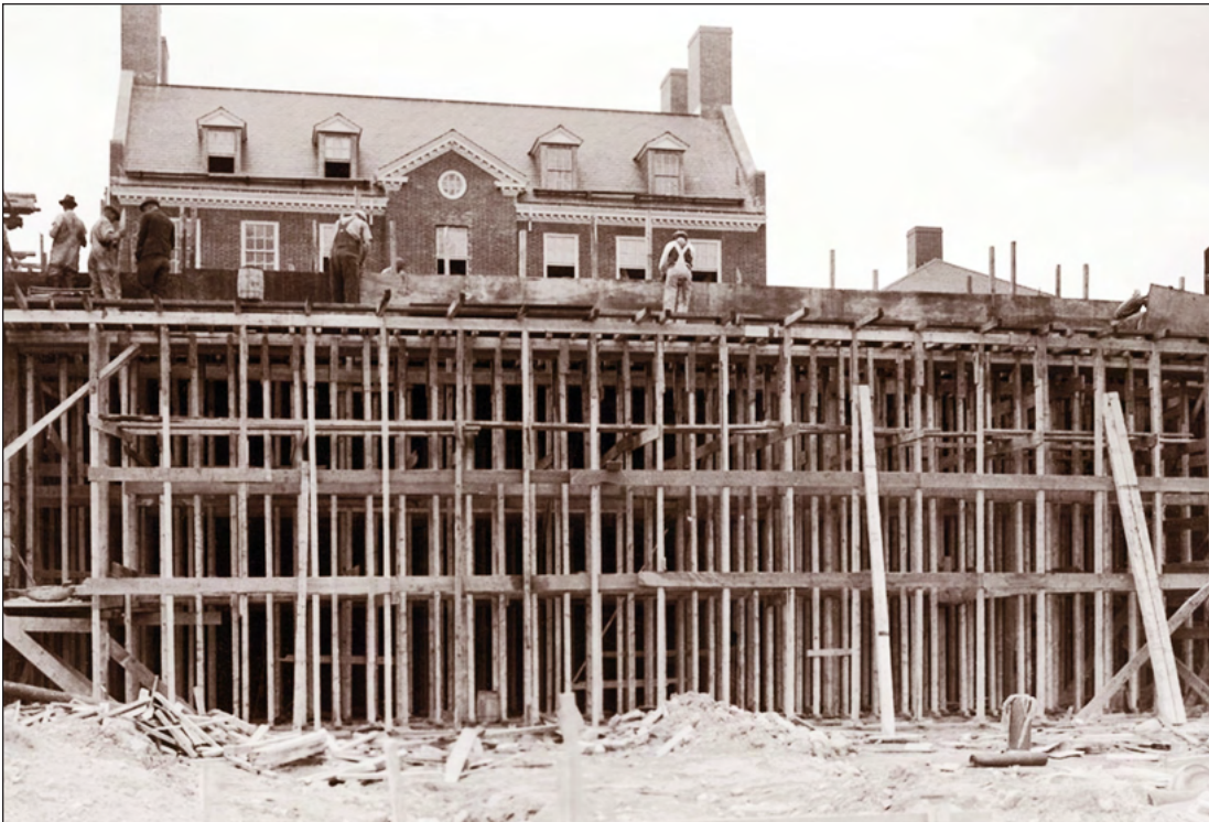
View of hangar under construction, 5-12-1938
