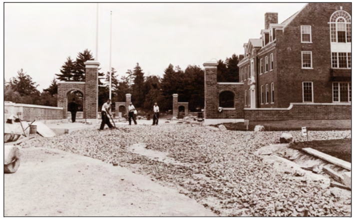
View of landscaping and brick arches - September 1938
