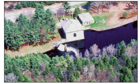
Aerial photo of Shaft 8 intake. DCR
