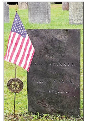
The Skinner gravestone after cleaning. The slight mottling is natural variation in the black slate.
