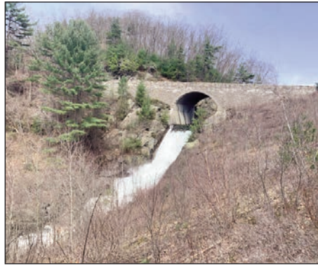
April 22, 2022 – Winsor Dam spillway
