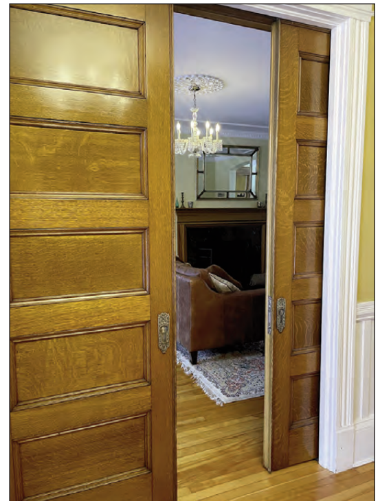
Pocket doors with ornate handles from the original Smith's Village house.
