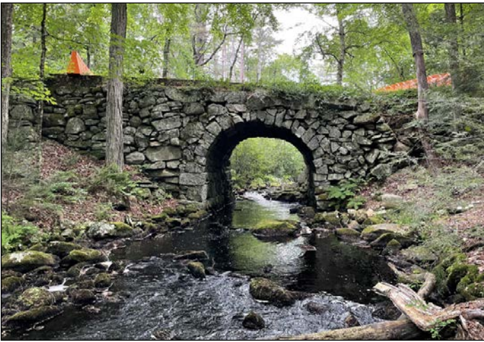
Arch ring showing flattening on south right side. -photo by Weitzner
