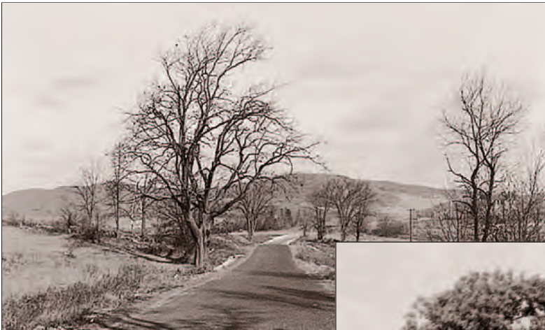
Around 1938 during reservoir construction.
