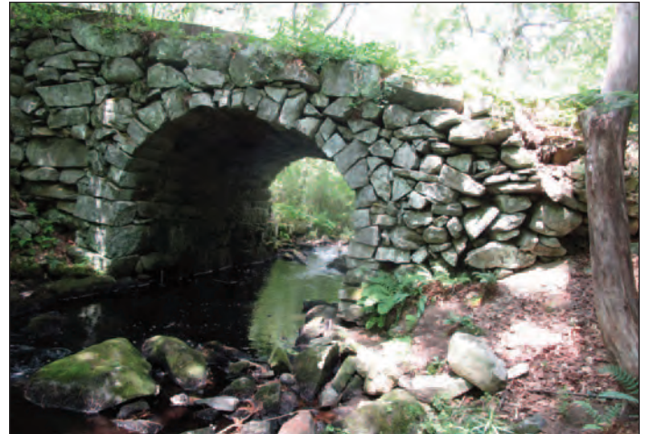
Keystone Bridge Collapse 2021
