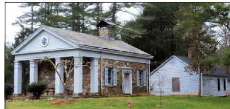
Quabbin Park Cemetery Administration Building and garage in rear
