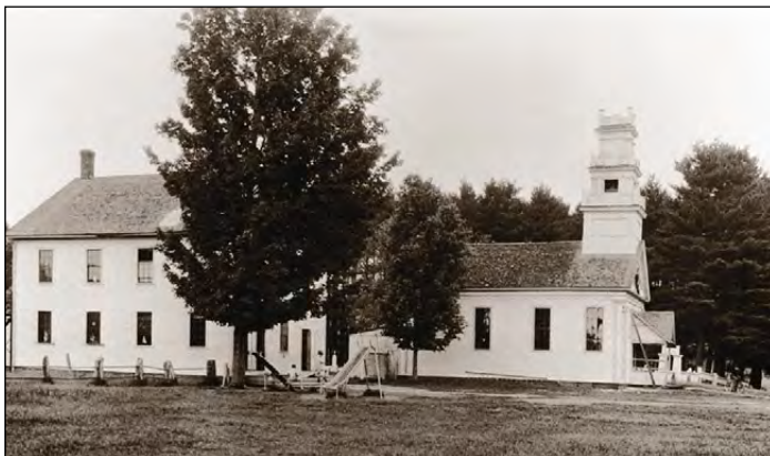
Dana Town Hall (right); School (left)
