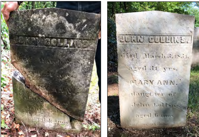
Left: Bob Howe holding the two fragmented pieces of the gravestone of his ancestor John Collins. Right: The repaired gravestone of John Collins. In addition to joining the two fragments together and filling the spaces and joints with the proper mortar, the gravestone was cleaned and treated with D/2 Biological Solution.
