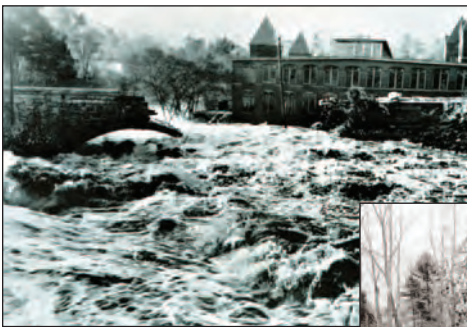
Bridge washout in Ware following 1938 hurricane
