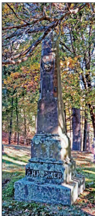
Left: H.H. Hosmer monument in Southwick's Old cemetery prior to cleaning with D/2 Biological Solution. You can easily see the built-up lichens and other biological growth. This monument is eleven feet tall.
