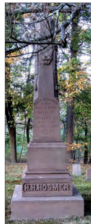
Left: H.H. Hosmer monument in Southwick's Old cemetery prior to cleaning with D/2 Biological Solution. You can easily see the built-up lichens and other biological growth. This monument is eleven feet tall.
