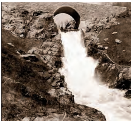
May 15, 1947 Quabbin spillway waterfall after Quabbin reaches 100% capacity
