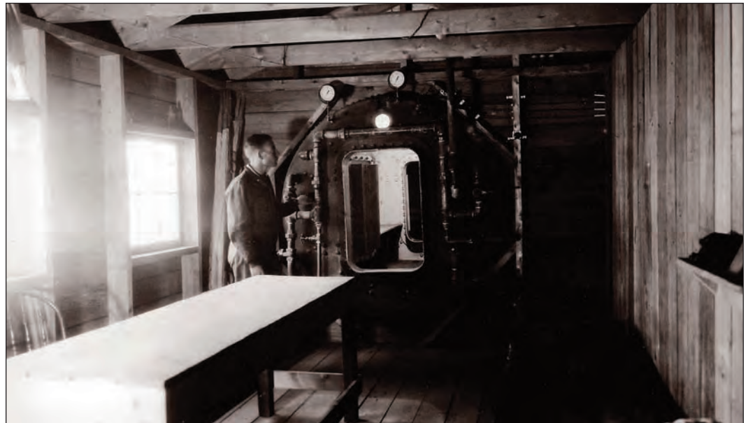
Photo of compression chamber. Was used for workers that worked in the caissons both at the dam and at the dike. Workers could only work for a period of 55 minutes in the caissons due to pressure.
