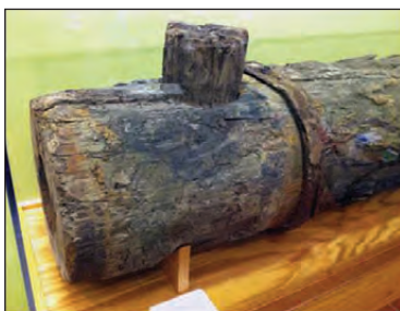
A wooden aqueduct with a fireplug from Boston’s early water system
