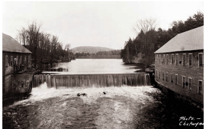
Dam at William Walker's Mills, April 25, 1928
