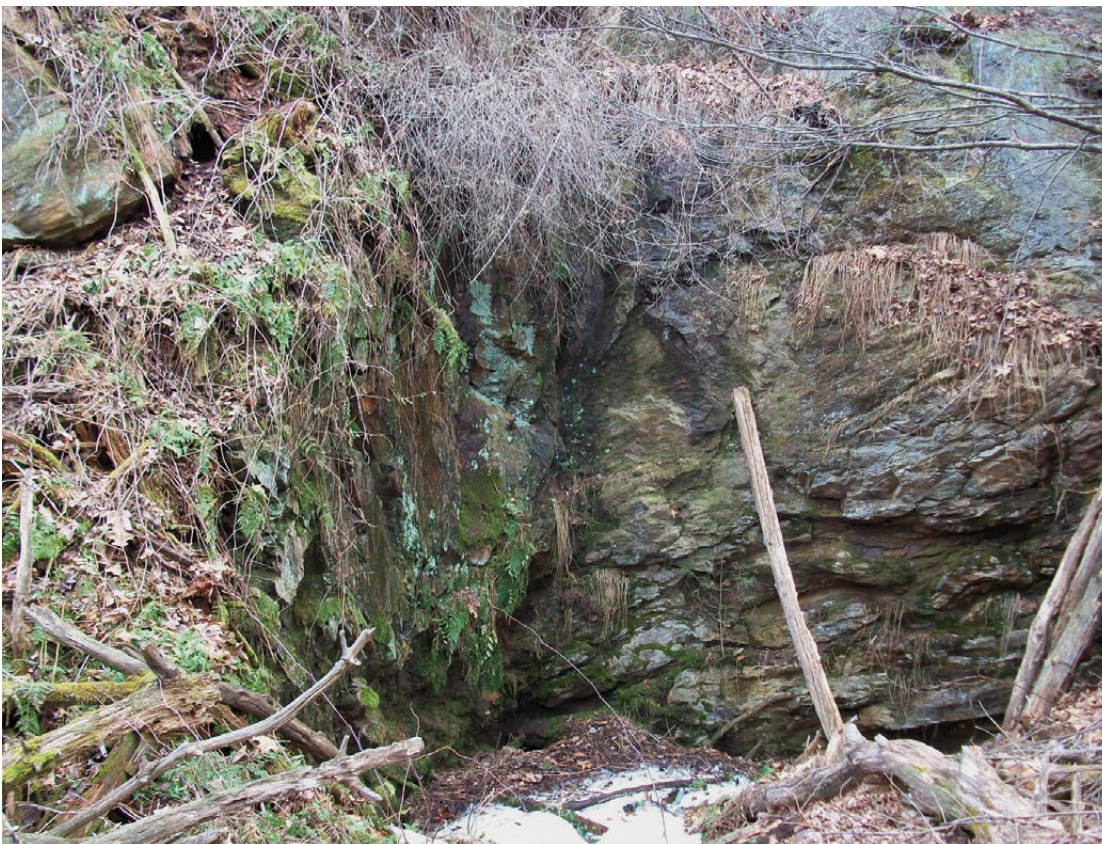
Photo by Stan Obrzut showing condition of the mine in 1981.
